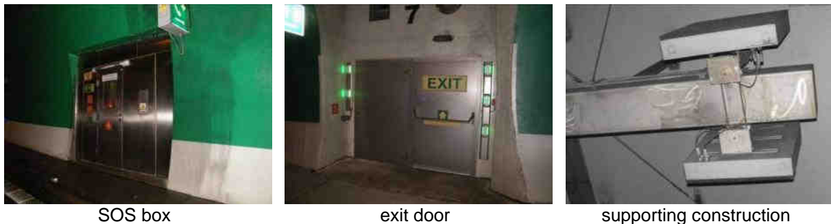
Figure 3: The examples of stainless steel application in the tunnel
