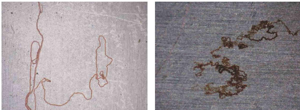
Figure 8: Examples of filliform corrosion on coupons
